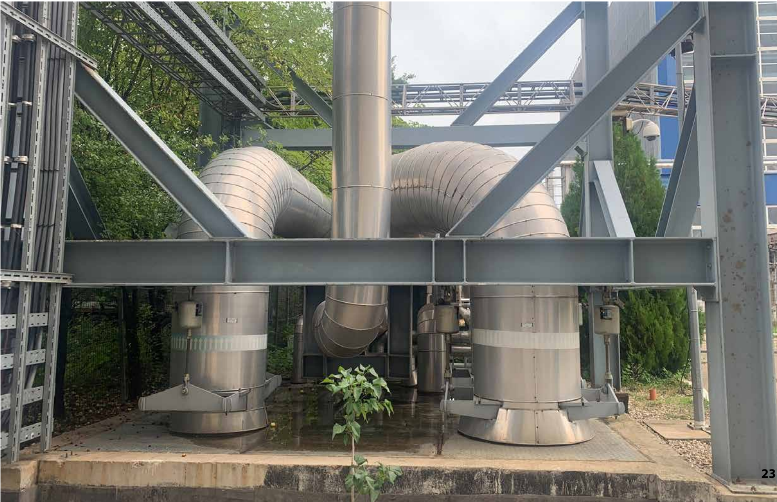
Thermal substation with heat exchangers to buildings. Photo by Shanti Pless, National Laboratory of the Rockies
